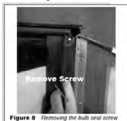
Figure 8 Removing the bulb seal screw
